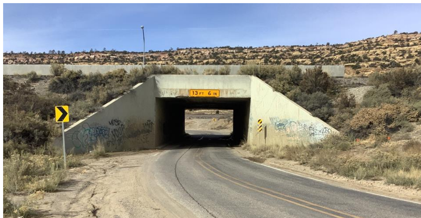
Exhibit 3-103. CBC (Bridge 6502) at MP 8.4, Height, and Width Restrictions
