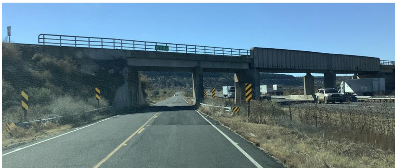
Exhibit 3-110. Narrow Roadway Width at MP 94.77, Bridge 6226 Due to Overhead Railroad Bridge
