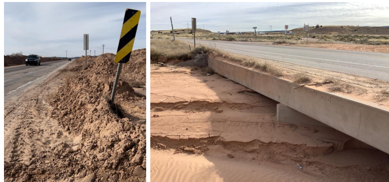
Exhibit 3-107. Clay Deposits from Severe Storm Events Covering the Drainage Structures
