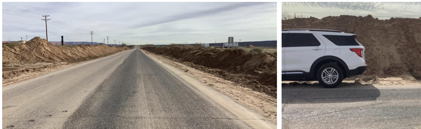
Exhibit 3-107. Clay Deposits from Severe Storm Events Covering the Drainage Structures
