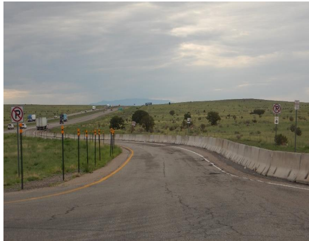
Signs, delineators, and concrete barriers prohibit truck parking on ramp.
