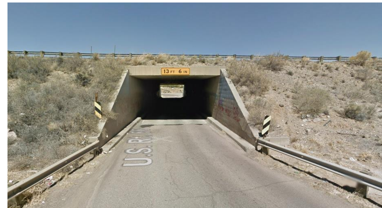
Exhibit 3-108. CBC (Bridge 6307) at MP 90.6, Height, and Width Restrictions
