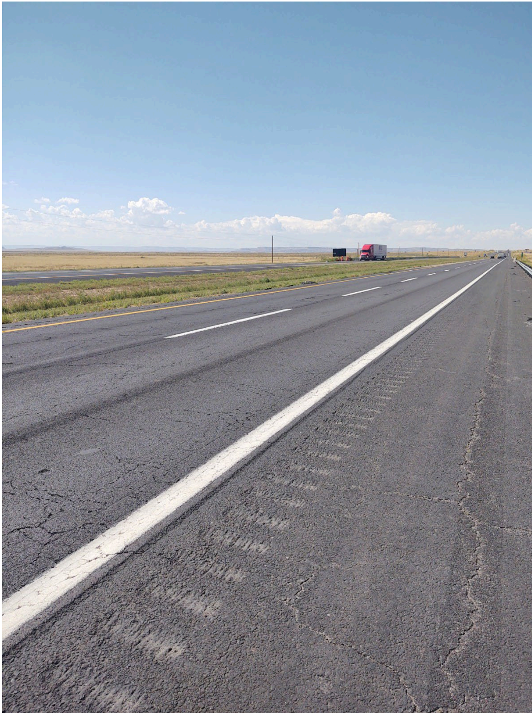
Photo 7: MP 126 - Looking SW along I-40
