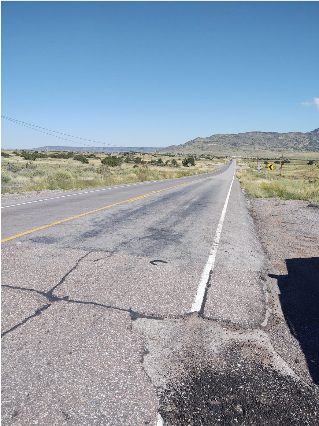
Photo 16: MP 90 - Looking W along Frontage Road
