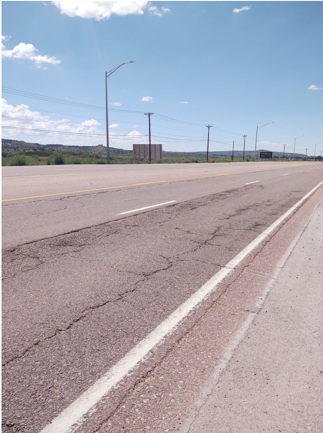
Photo 11: MP 18 - Looking SW along Frontage Road/Old Route 66
