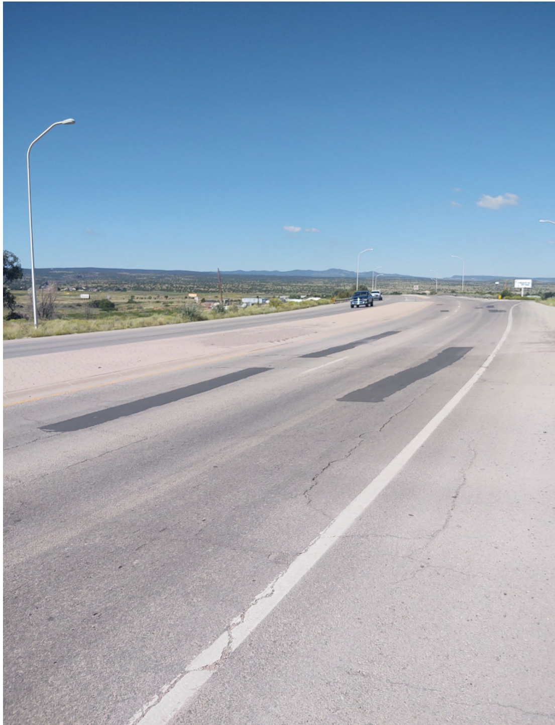
Photo 15: MP 80 - Looking W along Frontage Road
