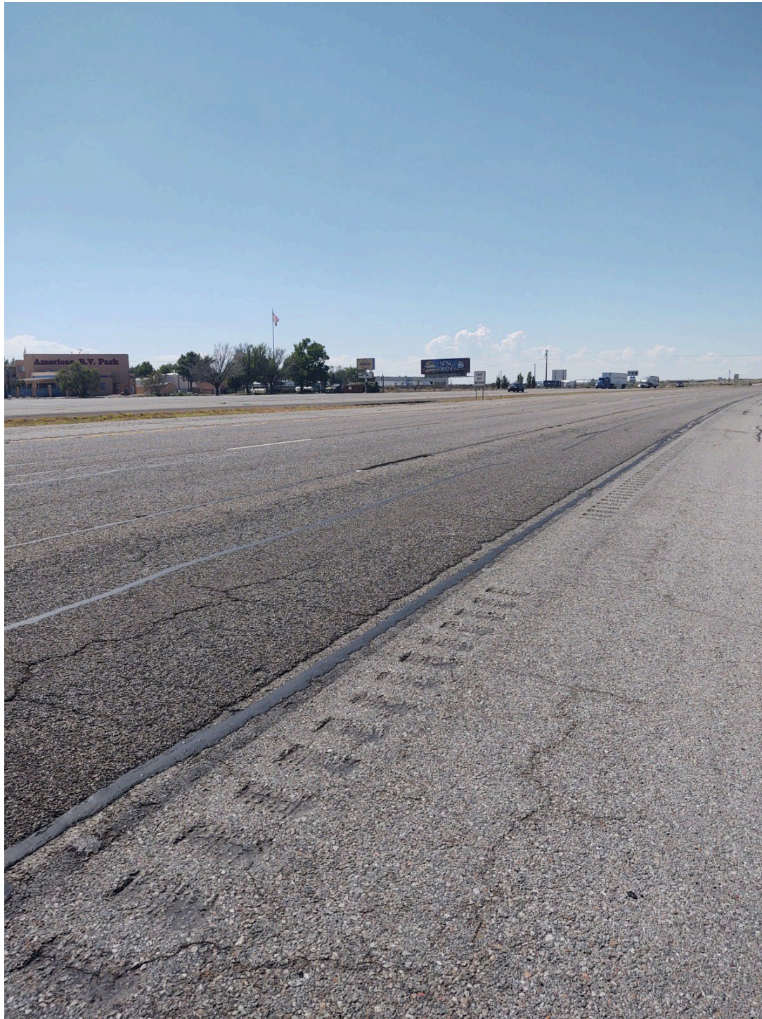
Photo 9: MP 149 - Looking SW along I-40
