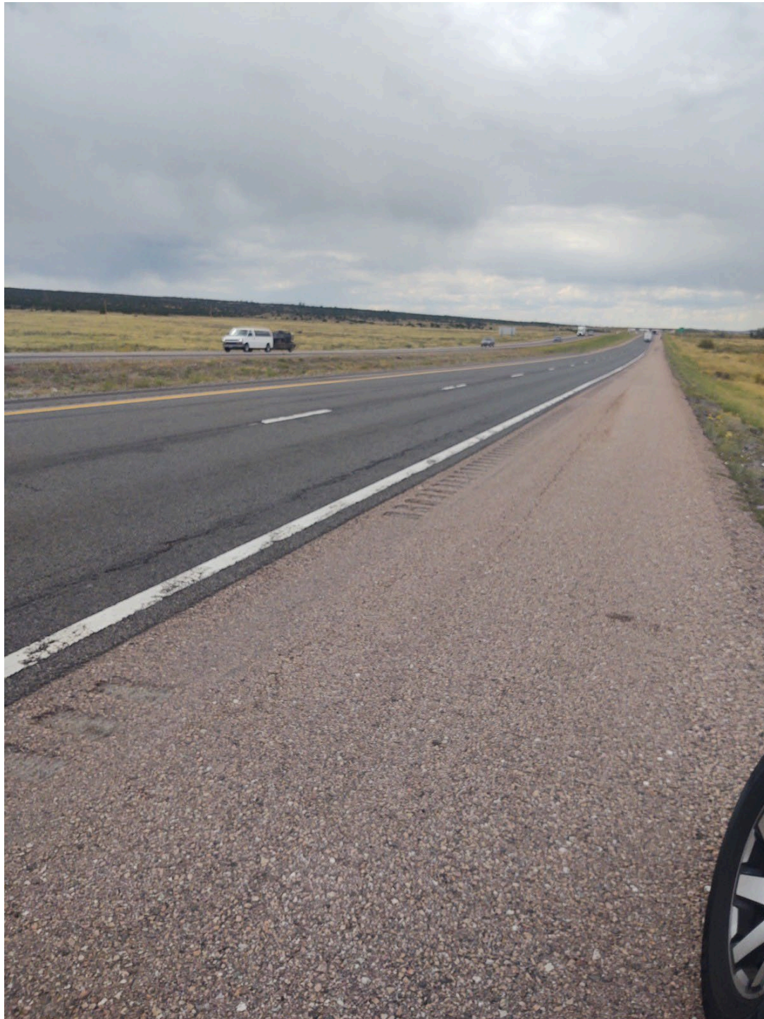
Photo 3: MP 38 - Looking SW along I-40
