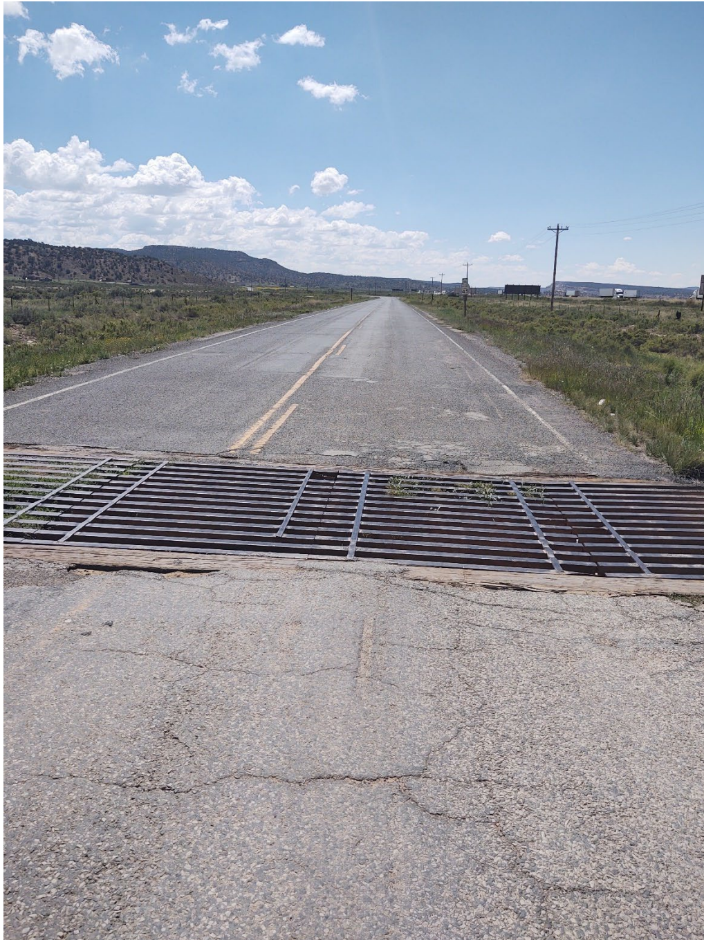
Photo 10: MP 7.5 - Looking W along Frontage Road
