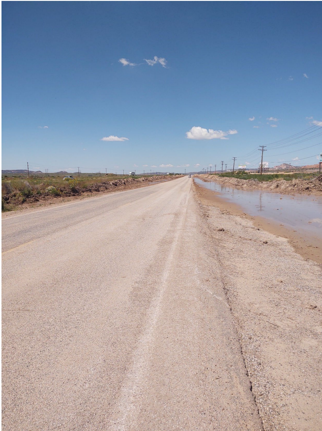
Photo 13: MP 33.5 - Looking W along Frontage Road
