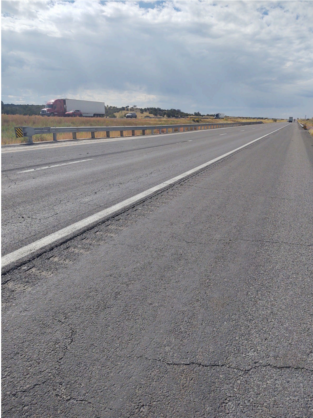
Photo 4: MP 58 - Looking SW along I-40
