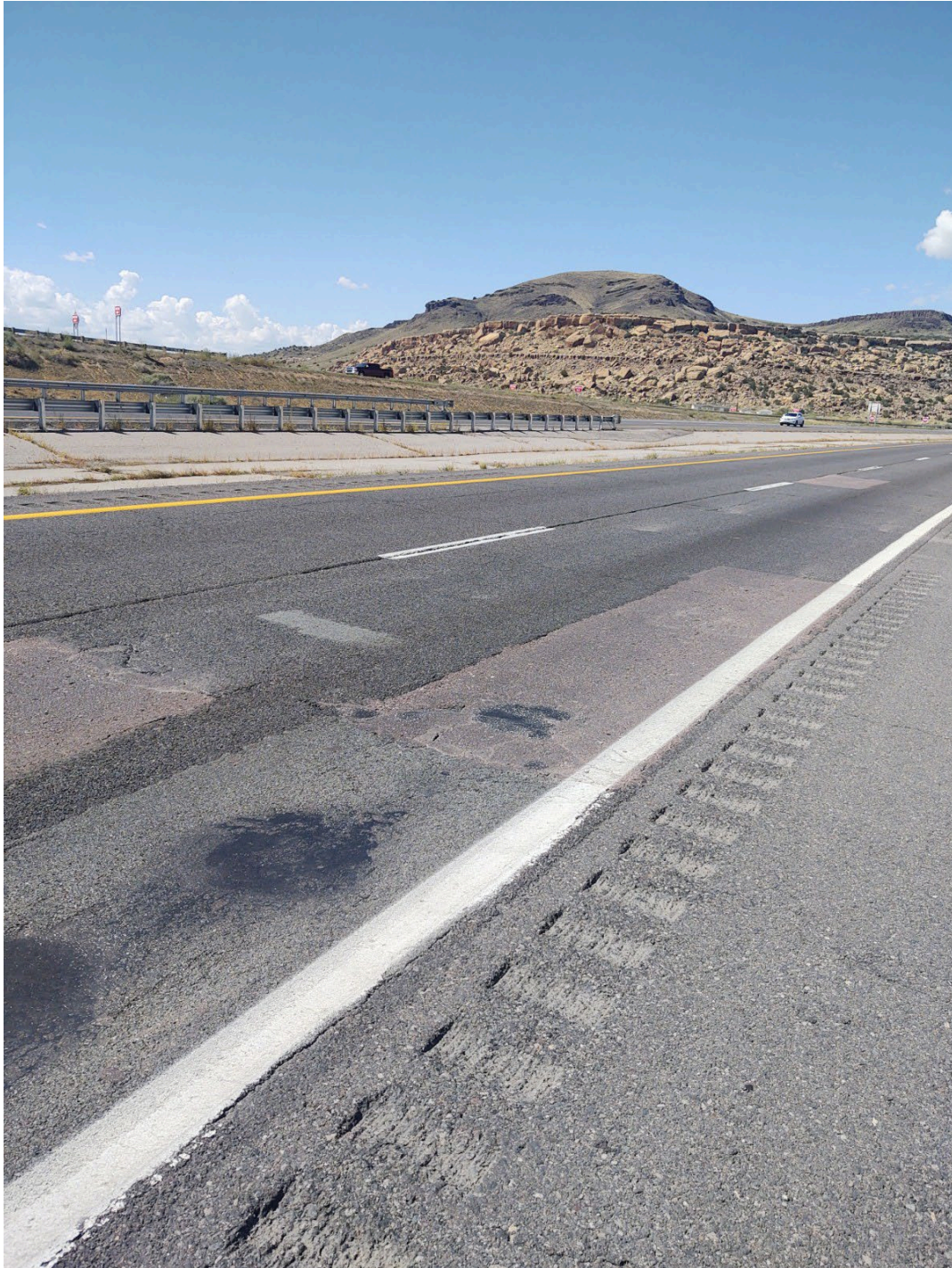
Photo 6: MP 104.5 - Looking NW along I-40
