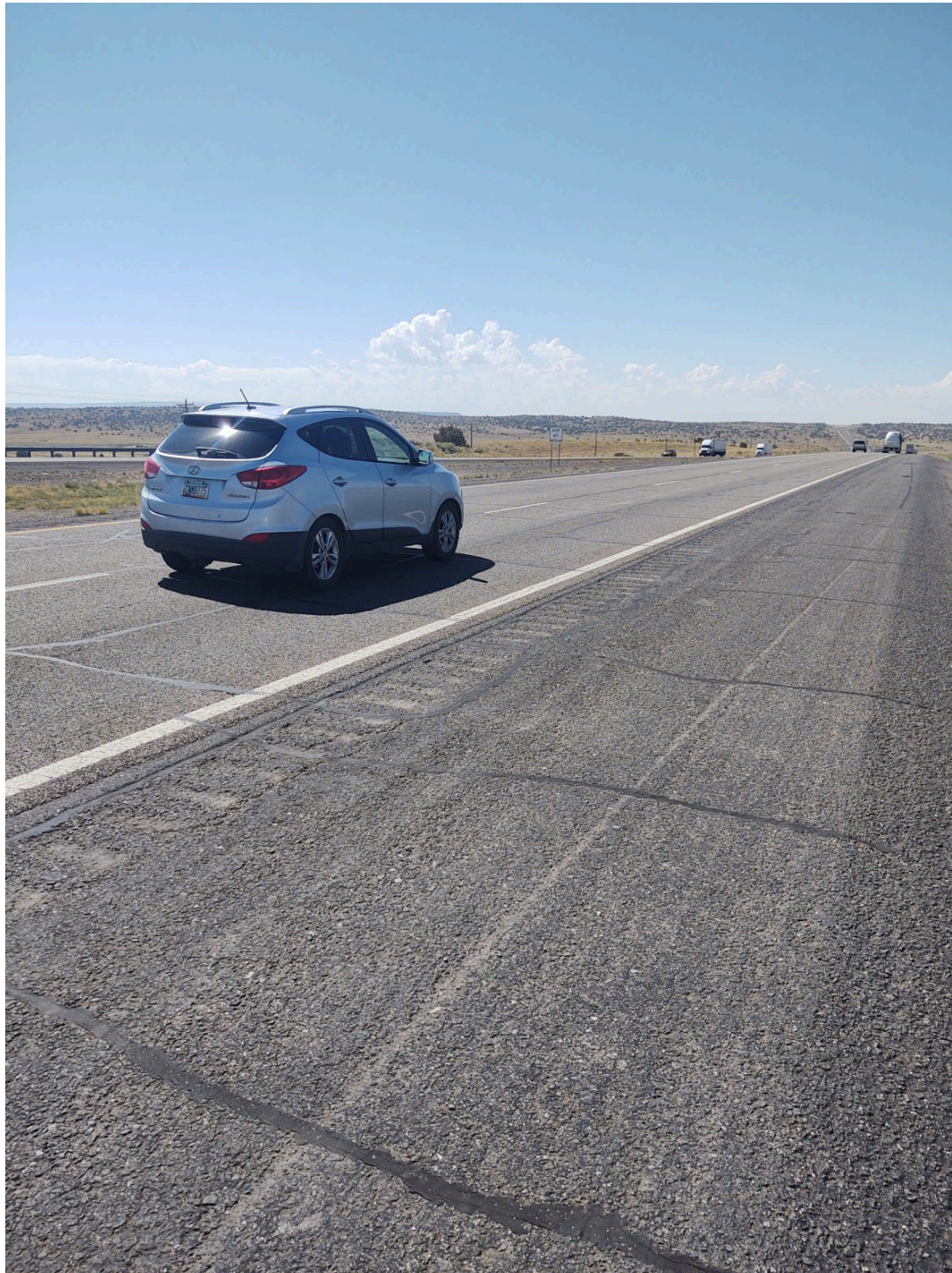
Photo 8: MP 138 - Looking SW along I-40
