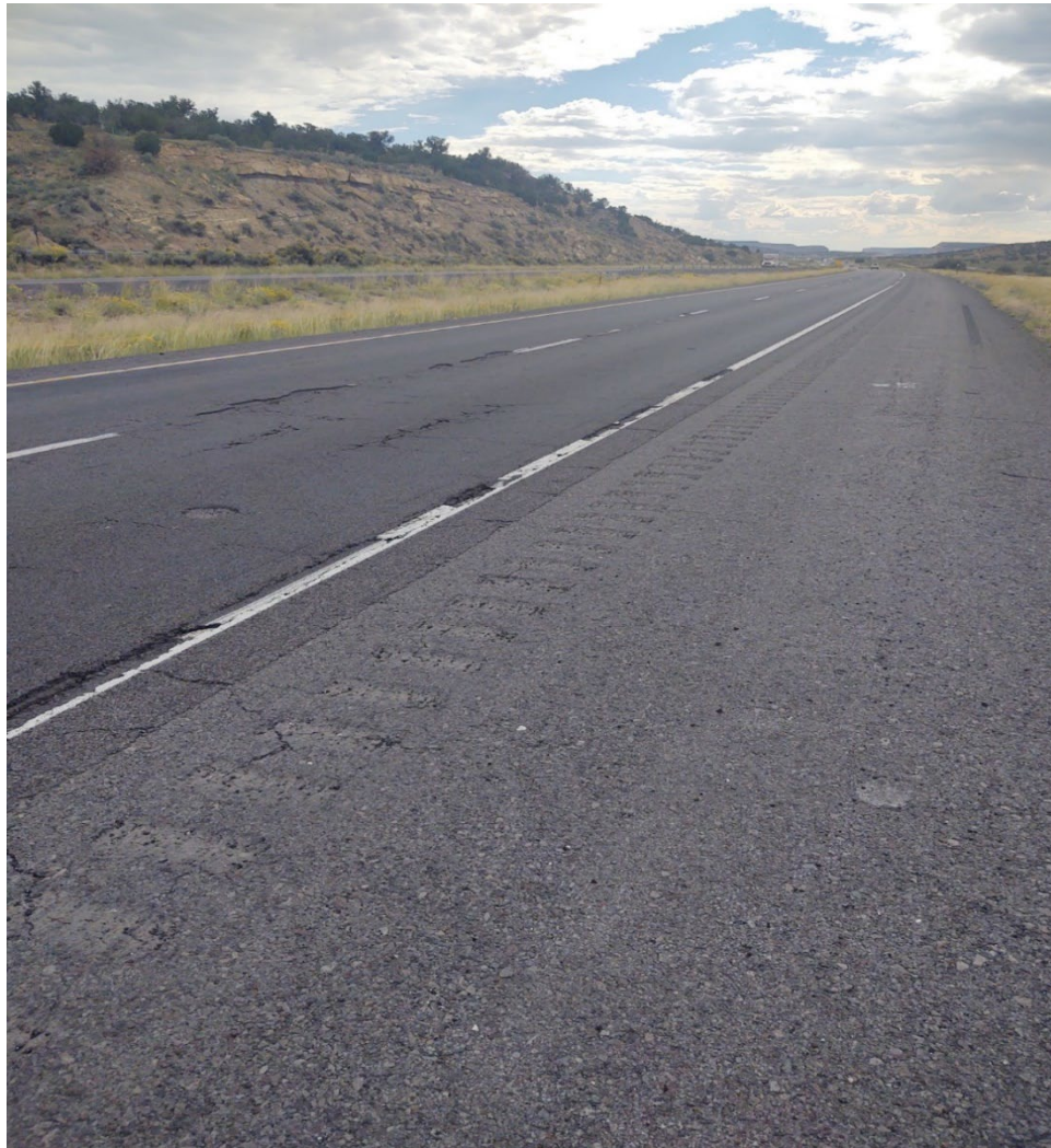
Photo 1: MP 10 - Looking West at WB Lane of I-40
