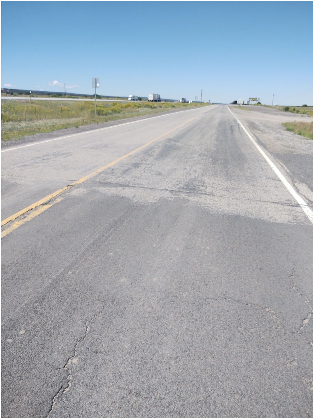
Photo 14: MP 52.5 - Looking W along Frontage Road
