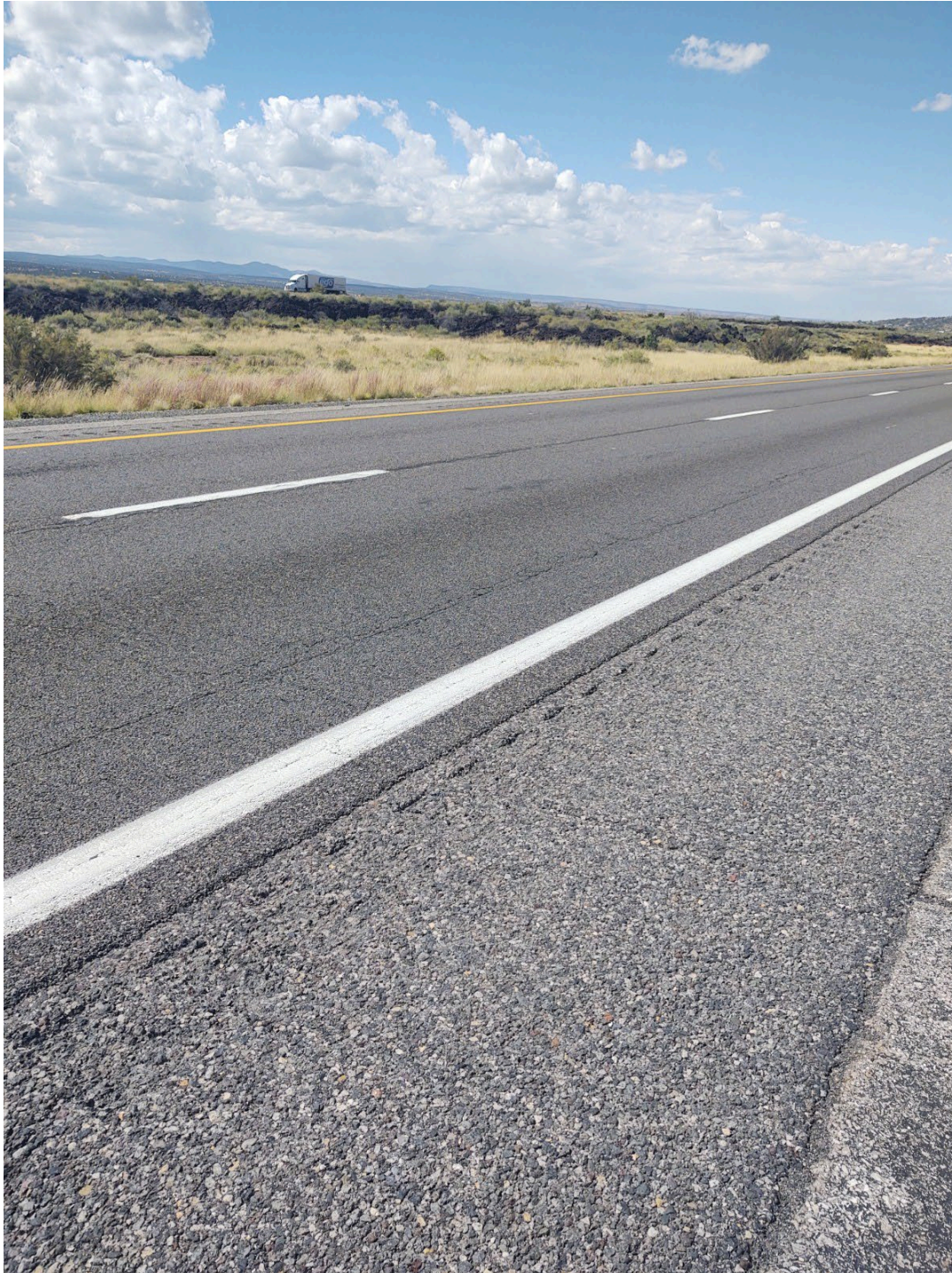
Photo 5: MP 84 - Looking W along I-40
