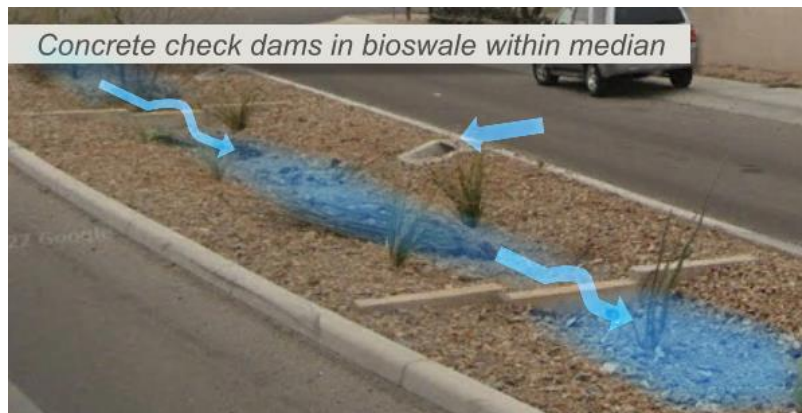
Figure 2: Example of Check Dams in a Roadway Median Bioswale
