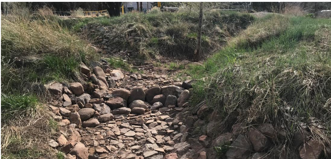
Figure 11: Example of a Rock Check Dam in a Bioswale Maintenance for Vegetation
