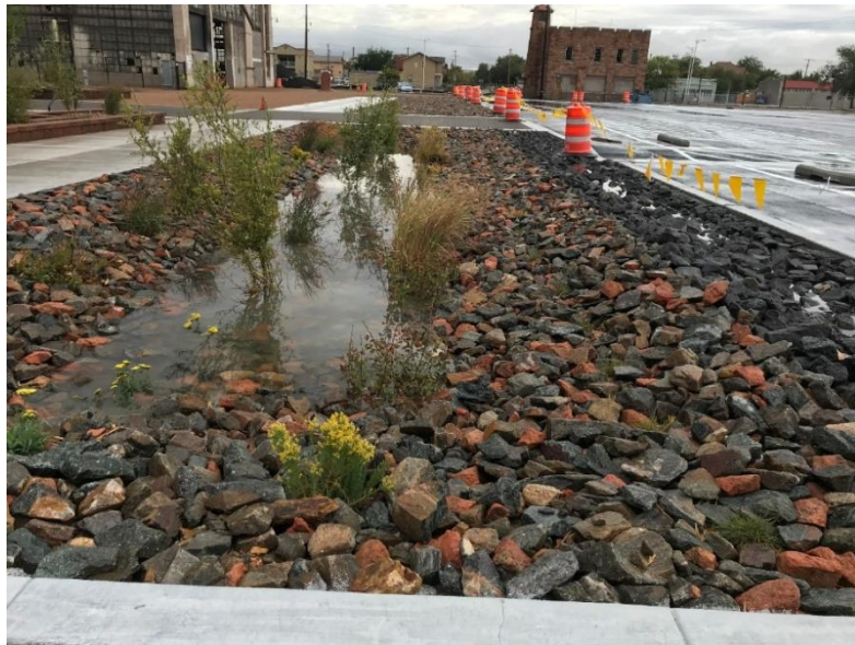
Figure 3: Example Stormwater Harvesting Basin (SHB)
