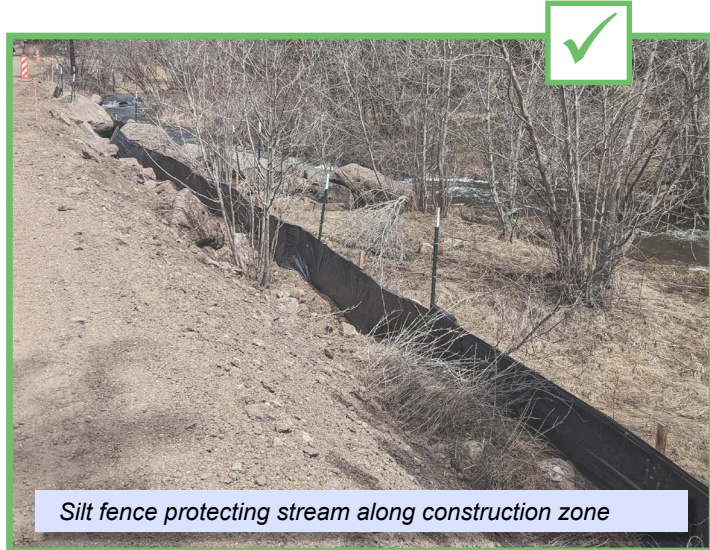
Excerpt of standard drawing or silt fence
