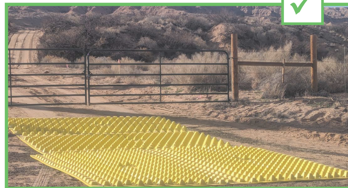
Track-out pad to trap construction sediment
