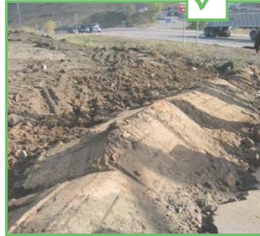
Compacted earth berm. Source: Minnesota Stormwater Manual
