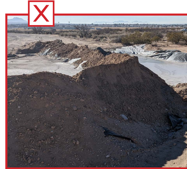
Earth berms with uncompacted soil would not withstand water flows or wind and can create an additional source of potential erosion and sediment.
