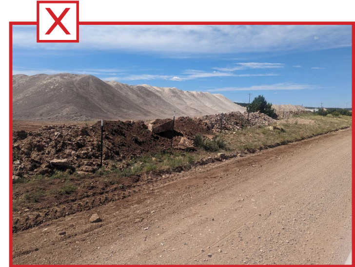
Earth berms with uncompacted soil would not withstand water flows or wind and can create an additional source of potential erosion and sediment.
