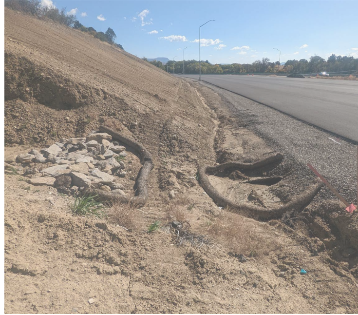
Correct: Rock check dam with mulch sock, mulch sock correctly located to protect culvert Incorrect: Unstabilized slope, sediment collected at culvert, mulch socks not staked and overlapping mulch socks Incorrect: Rock check dam with mulch sock, mulch sock correctly located to protect culvert may have been added after culvert filled with sediment, roadside ditch may need check dam
