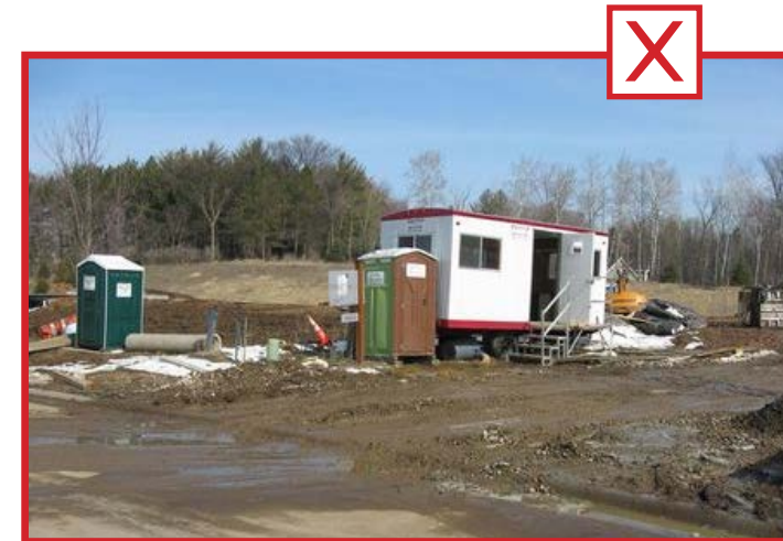
No sediment control at entrance/ exit, sediment tracked off-site. Source: Minnesota Stormwater Manual
