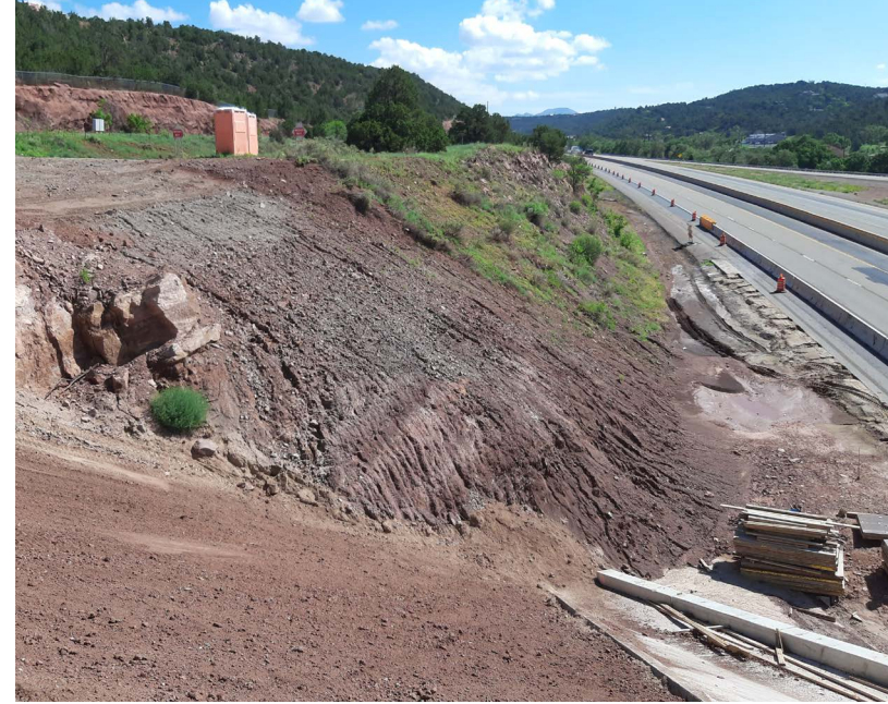
Correct: Port-a-potties located away from flow paths Incorrect: Unstabilized slope, rilling along roadway, visible tracking in collected sediment, materials stockpiled within flow path
