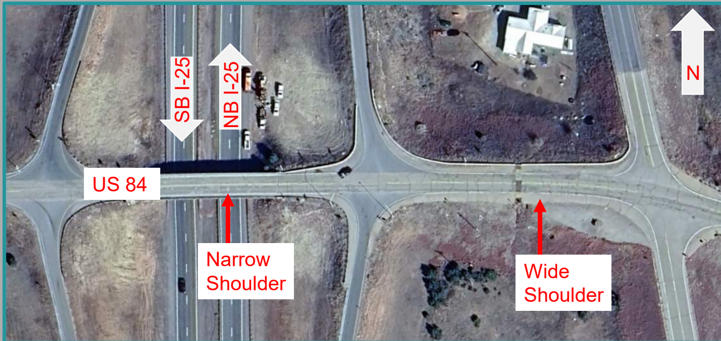
Aerial View of Project Area Showing Varying Shoulder Widths on US 84
