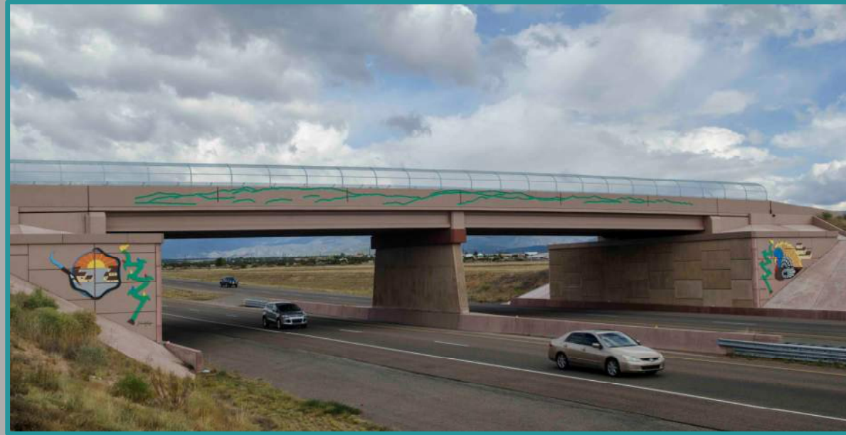
Example of Bridge Artwork
