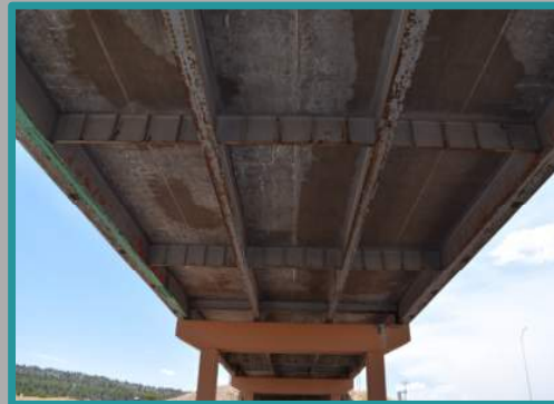
Concrete Deterioration and Corrosion of Steel Members
