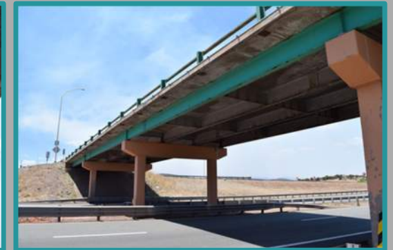
Concrete Deterioration and Corrosion of Steel Members
