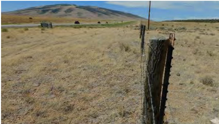
Figure D-10. Lay-down fence in erect setting on the Rio Grande Del Norte National Monument, Tres Piedras, New Mexico (photo credit: P. Cramer).
