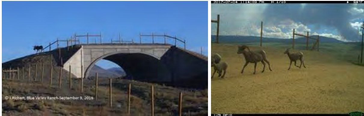
Figure D-14. Moose used the Colorado SH 9 overpass the first fall after completion (left). The overpass was created with pre-fabricated arches (photo credit: J. Richert, Blue Valley Ranch). Bighorn sheep use a Colorado SR 9 overpass (right) (photo credit: Eco-Resolutions, CDOT, and CPW).
