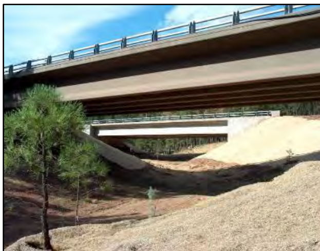
Figure D-21. In Arizona, SR 260 wildlife crossing bridges were found to facilitate over 6,000 successful elk crossing movements (Gagnon et al., 2011) (photo credit: AZGFD).
