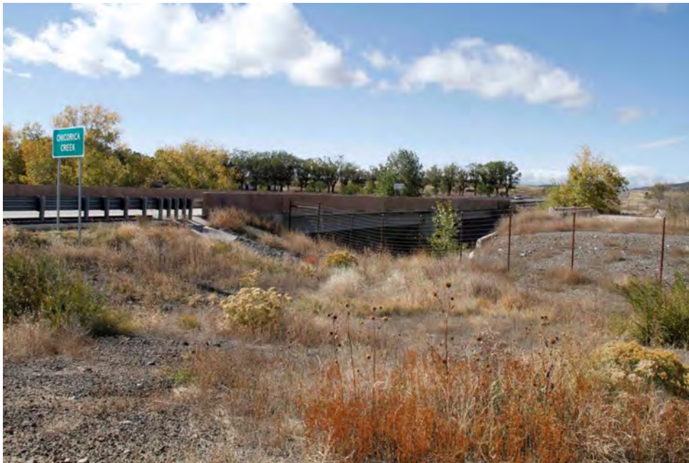
Figure 1-4. A small fencing project implemented in 2004 to mitigate a relatively high deer-vehicle collision hotspot along US 64 in northeastern New Mexico between Raton and Clayton. Chicorica Creek contains riparian vegetation and perennial water in shortgrass prairie habitat. A 0.1-mile game fence was constructed on each end of a bridge that was enlarged during the US 64 highway improvement project (photo credit: Mark Watson).
