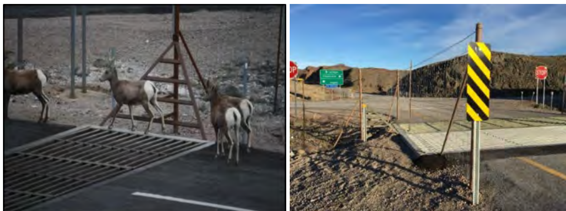
Figure D-44. Desert bighorn sheep breach a single cattle guard by using support lip in Arizona (left). The guard was adapted to a double cattle guard and the vault lip was covered with fence (right). Monitoring Found no bighorn sheep breaches after retrofit (photo credit: AZGFD, AZDOT).
