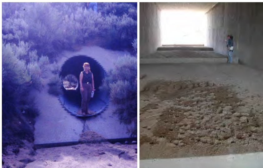
Figure D-12. US 550 original corrugated metal culvert (left), replaced with a wildlife crossing concrete box culvert (right) in the Aztec Project (photo credit: M. Watson).
