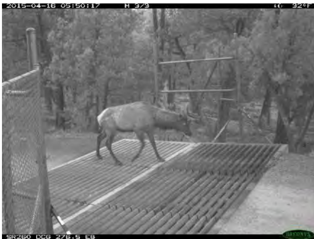
Figure D-42. Elk breaches double cattle guard in Arizona (photo credit: AZGFD and AZDOT).
