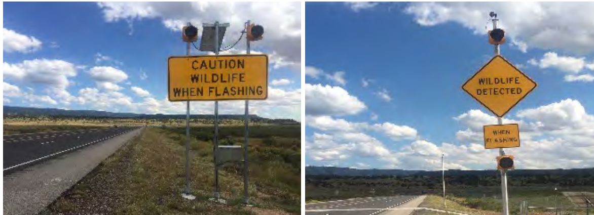
Figure D-57. Wildlife activated driver warning system on US 550, New Mexico (photo credit: AZGFD).
