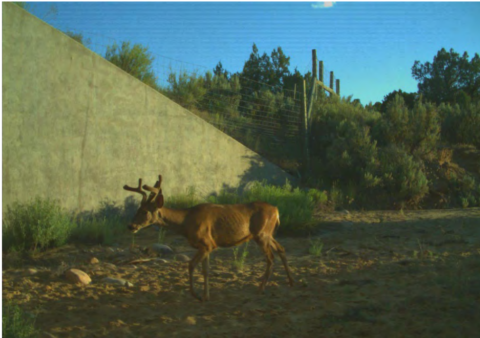
Figure A-24. Mule deer buck using concrete box culvert to move beneath US 550 (photo credit: AZGFD, NMDOT).
