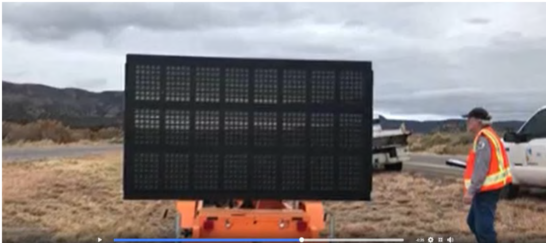
Figure A-3. Installation of driver warning variable message board along US 70.
