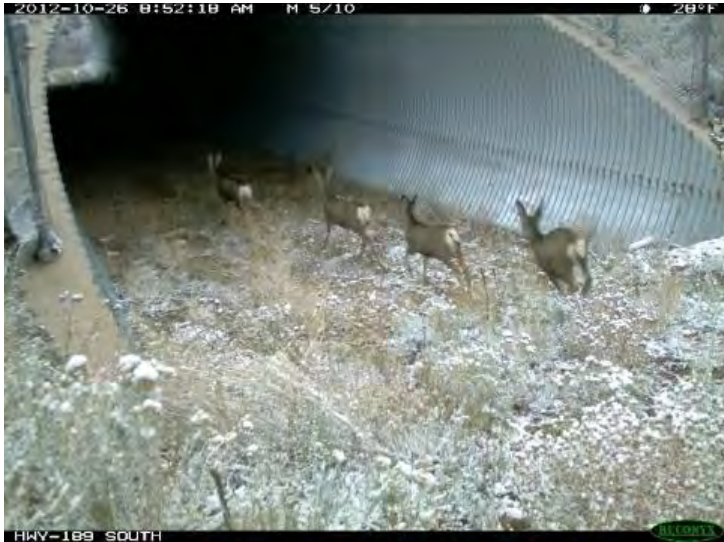
Figure D-32. In Utah, mule deer use a large corrugated steel culvert underpass in Deer Creek State Park under US 189 (photo credit: P. Cramer, UDOT).
