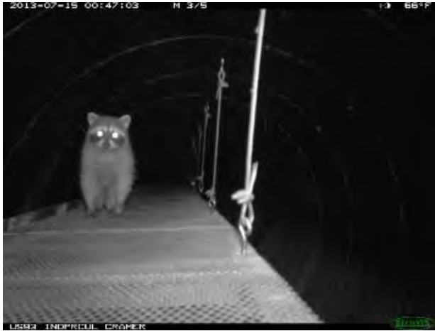
Figure D-3. Small mammal shelf placed in a Montana culvert facilitated movement of raccoons and other wildlife (photo credit: P. Cramer and Montana DOT).
