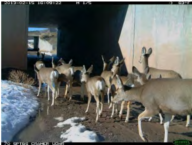
Figure D-28. In Utah, once wildlife exclusion fence was placed along this USFS road that encompassed a pair of concrete box culverts, mule deer began using these to pass beneath I-70, with hundreds of successful mule deer movements through the pair of culverts each year (Cramer, 2012 and 2014) (photo credit: P. Cramer, UDOT, and UDWR).
