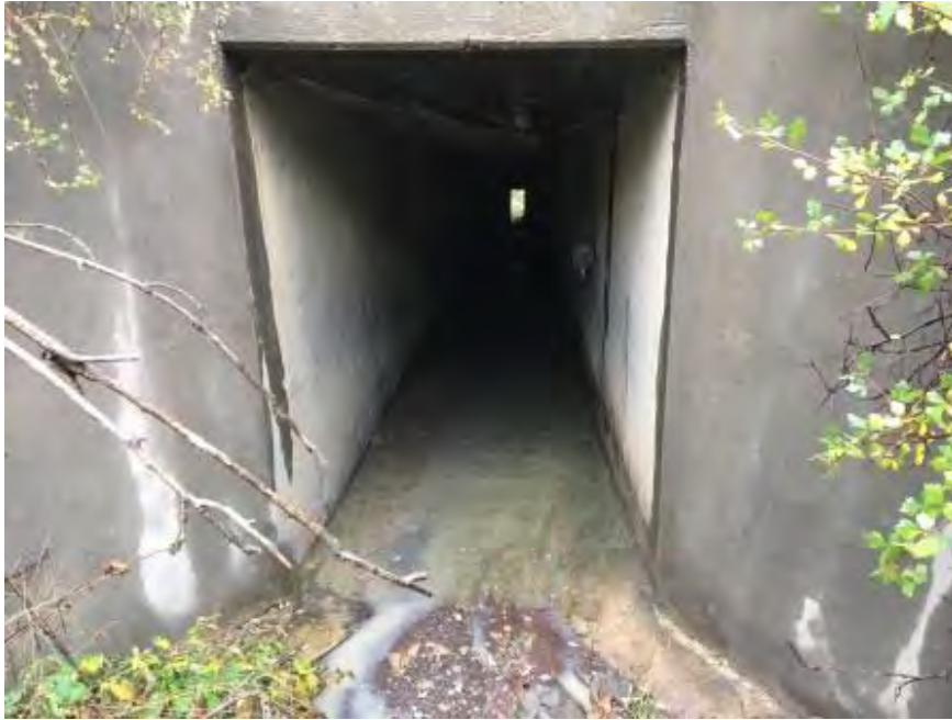
Figure A-11. I-25 Raton Pass MP 458.1 box culvert (photo credit: AZGFD).
