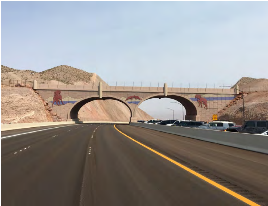
Figure 1-6. Desert bighorn sheep overpass built during Phase II of the I-11 Boulder City Bypass mitigation project in southeastern Nevada (photo credit: Jeff Gagnon).
