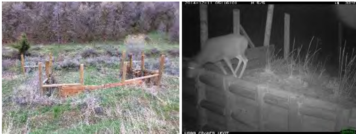
Figure D-38. A Utah high migration escape ramp on US 91 (left). Three sides provide three escape opportunities (photo credit: P. Cramer). Mule deer uses a high migration escape ramp in Utah, US 91 (right) (photo credit: P. Cramer, UDOT).
