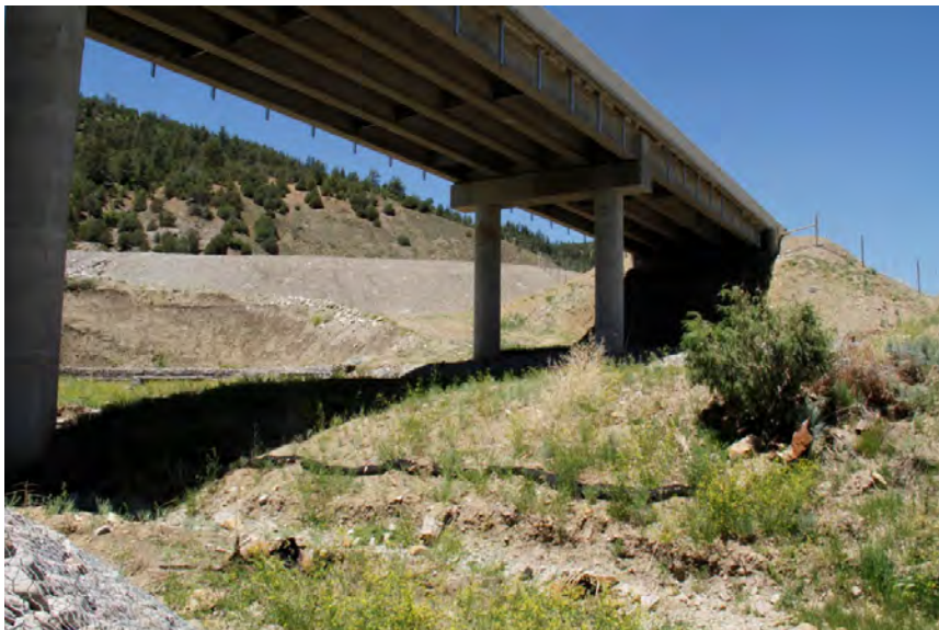
Figure A-19. US 64 near Lumberton Bridge over Amargo Creek at MP 144.8.
