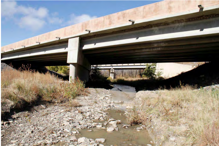
Figure A-14. US 54 Bridge at Chicorica Creek
