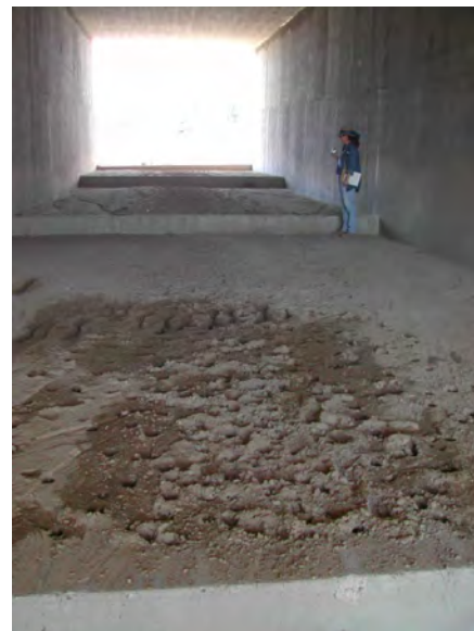
Figure A-22. US 550 original corrugated metal culvert (left) replaced with a wildlife crossing concrete box culvert (right) in Aztec Project (photo credit: M. Watson).
