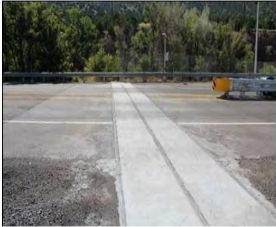
Figure D-59. Tijeras Canyon Safe Passage Project electrified concrete barriers at NM 333 wildlife crosswalk (photo credit: AZGFD).
