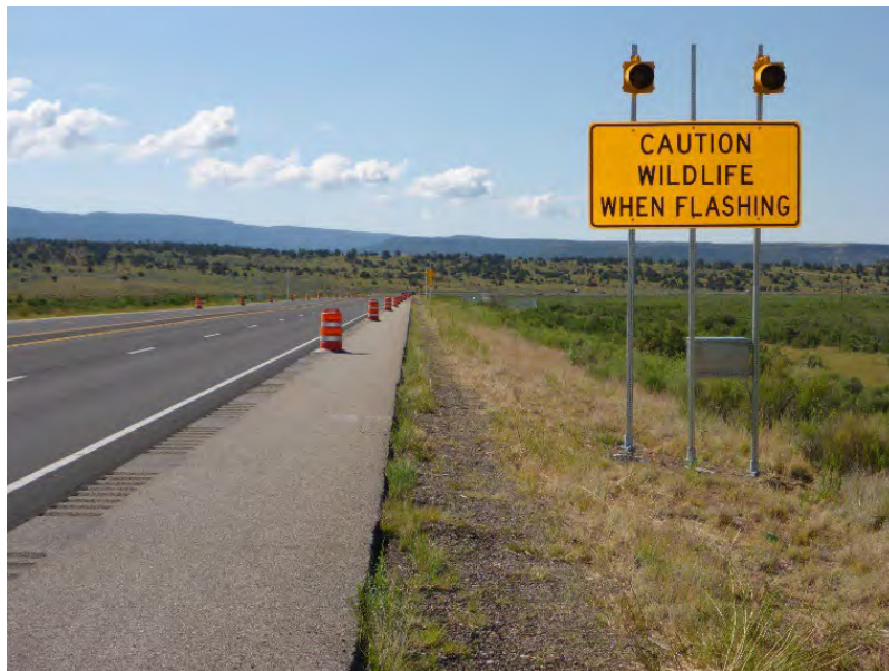
Figure A-26. Wildlife-activated driver warning system on US 550 (photo credit: NMDGF, NMDOT).
