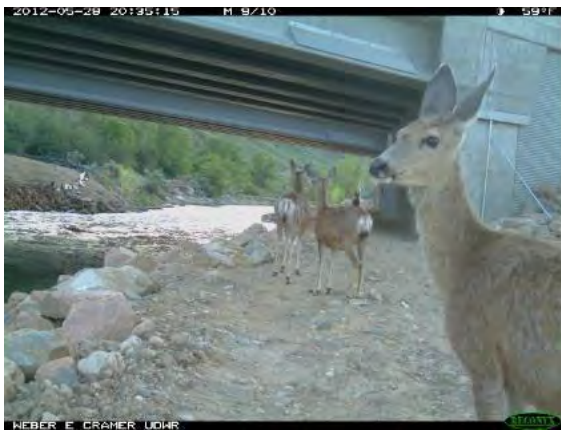
Figure D-20. In Utah, mule deer use wildlife crossing bridge at the Weber River, under I-80 (photo credit: P. Cramer, UDOT, UDRW).
