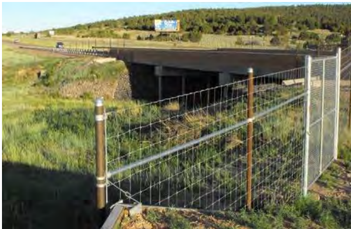
Figure D-1. Bridge under I-40 that wildlife use near Edgewood, New Mexico. Mule deer and other wildlife are directed to the area under the bridge for movement beneath I-40 (photo credit: M. Watson and J. Hirsch).
