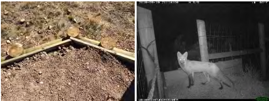
Figure D-37. Angle of escape ramp in fence along Utah’s US 189 (left). Red fox on Utah escape ramp on US 189 (right). Ramp is at approximately a 150 degree angle to fence line (photo credit: P. Cramer, UDOT).
