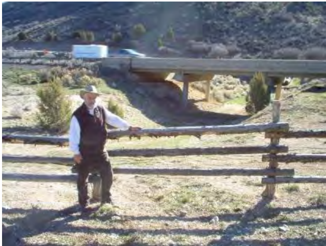
Figure D-34. Utah wildlife rail fence at a wildlife crossing structure under I-15 (photo credit: P. Cramer).
