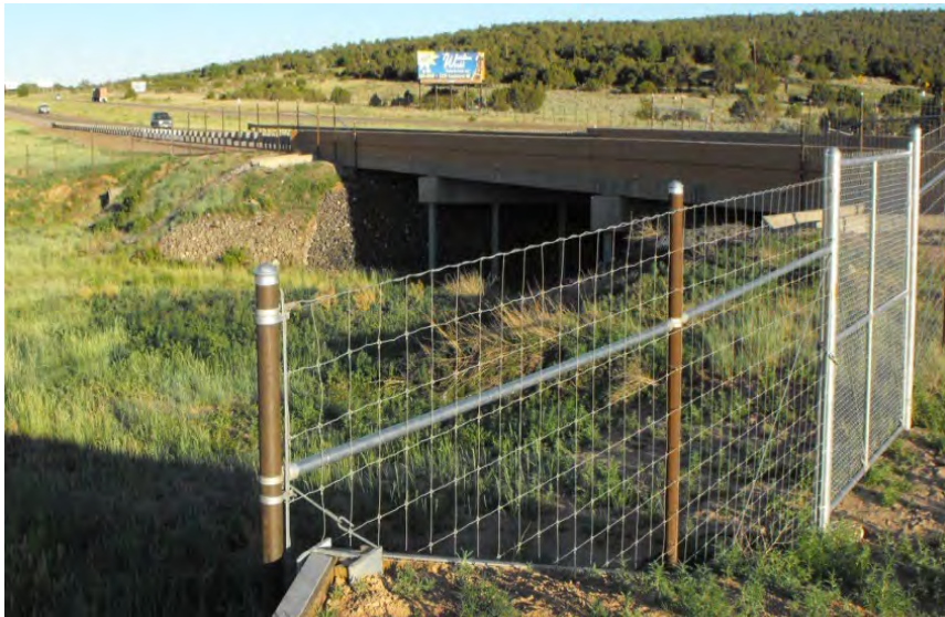
Figure A-7. Bridge under I-40 used by wildlife near Edgewood (photo credit: M. Watson).
