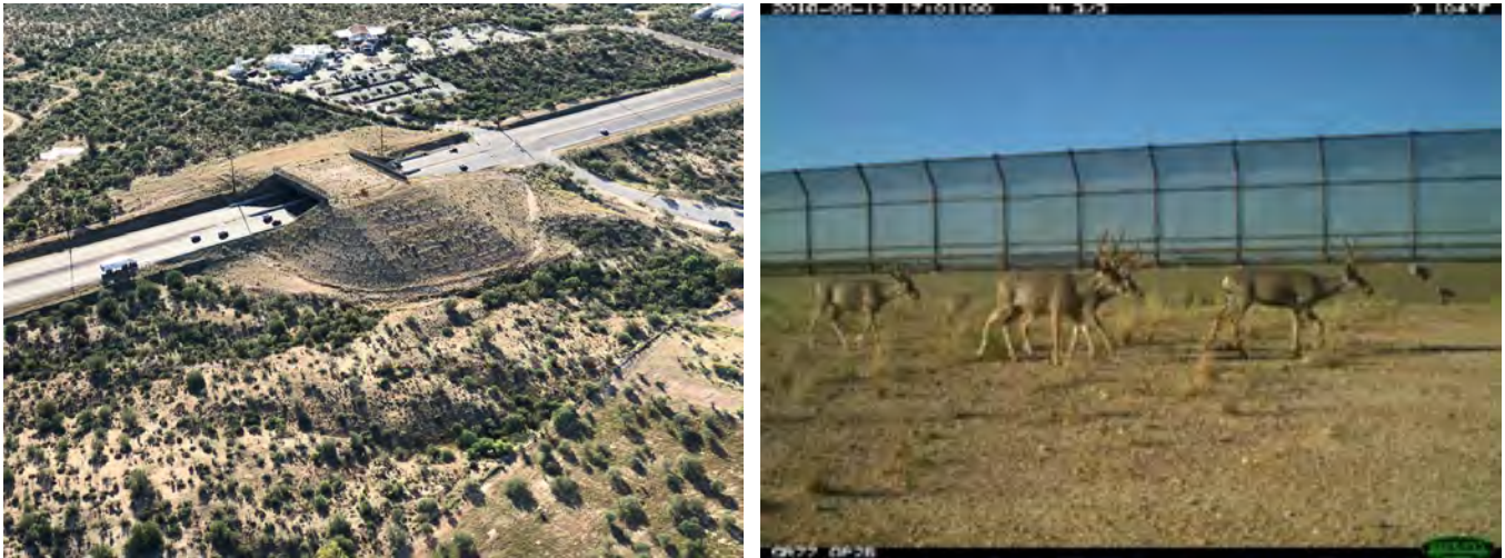
Figure 1-9. First wildlife overpass in the Sonoran Desert along State Route 77 in southern Arizona (photo credit: AZGFD).
