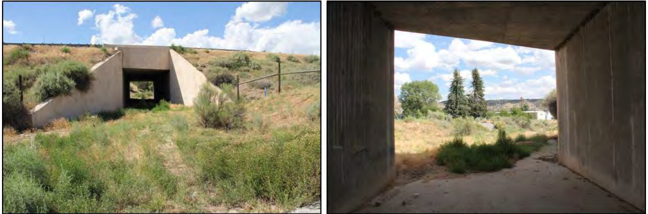
Figure A-23. US 550 wildlife crossing concrete box culverts (photo credit: AZGFD).
