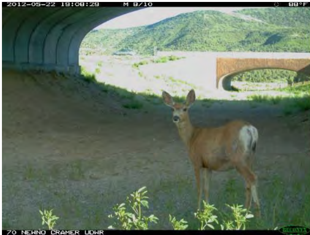
Figure D-24. Mule deer used the arch underpass under I-70 in Utah (photo credit: P. Cramer, UDOT, and UDWR).
