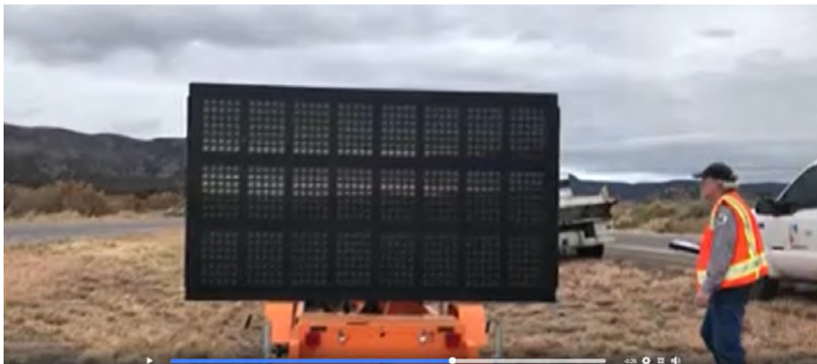
Figure 6-25. M. Watson of NMDGF together with NMDOT maintenance personnel, installed a driver-warning variable message board on US 70 in the wildlife-vehicle hotspot (photo credit: NMDGF).
