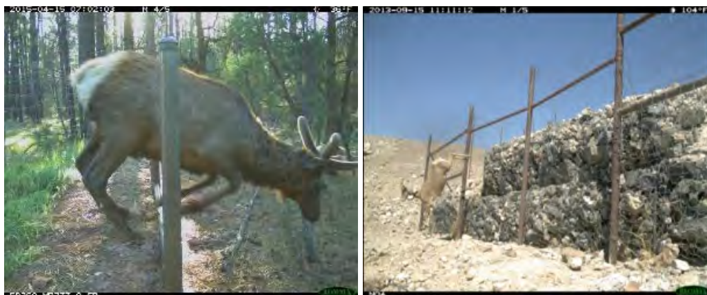
Figure D-39. Elk use escape ramp (left) and desert bighorn sheep use a 6-foot escape ramp (right), both in Arizona. The bar on the desert bighorn ramp was placed higher than 6 feet (photo credit: AZGFD and AZDOT).
