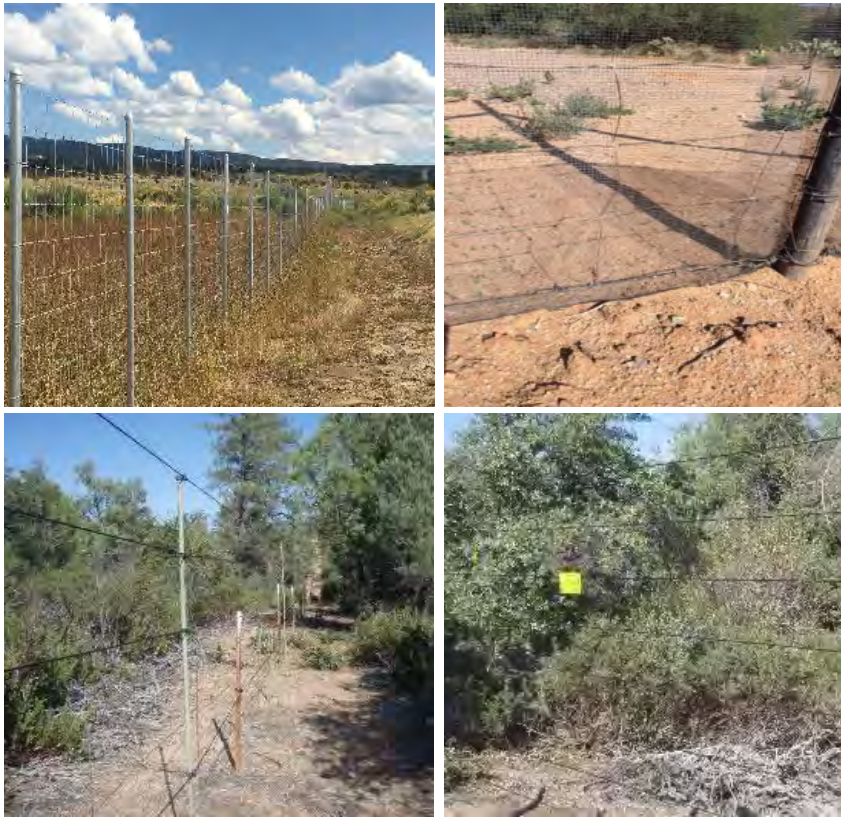
Figure D-33. Traditional field fence 8 feet high (top left), woven wire mesh fence for smaller wildlife (top right), standalone electrified braid fence (bottom left), and combination of electrified braid and standard right of way fence to limit elk access to Arizona’s SR 260 (bottom right) (photo credit: AZGFD).
