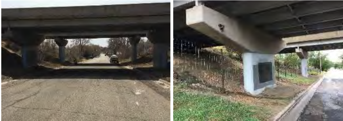
Figure D-5. New Mexico I-25 Raton Interchange where retrofit fence was added and existing pathways were available and used by wildlife (photo credit: J. Gagnon, AZGFD).
