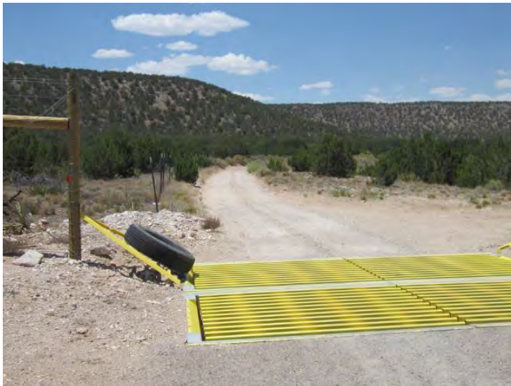
Figure A-2. US 54 double cattle guard with wing and tire to prevent wildlife from walking across the guard (photo credit: Mark Watson).
