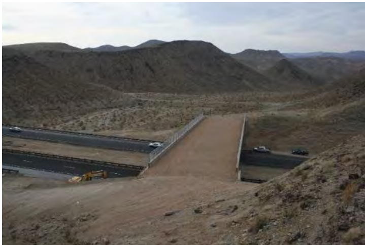
Figure D-18. Arizona US 93 desert bighorn overpass (photo credit: AZGFD).
