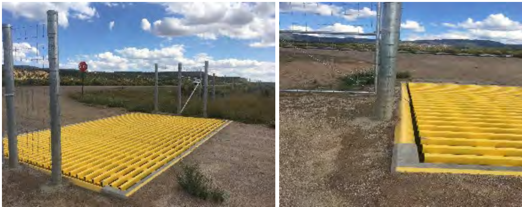
Figure D-46. In New Mexico, US 550 Cuba double-width game (cattle) guard with perpendicular fence and beveled vault edges (photo credit: AZGFD).
