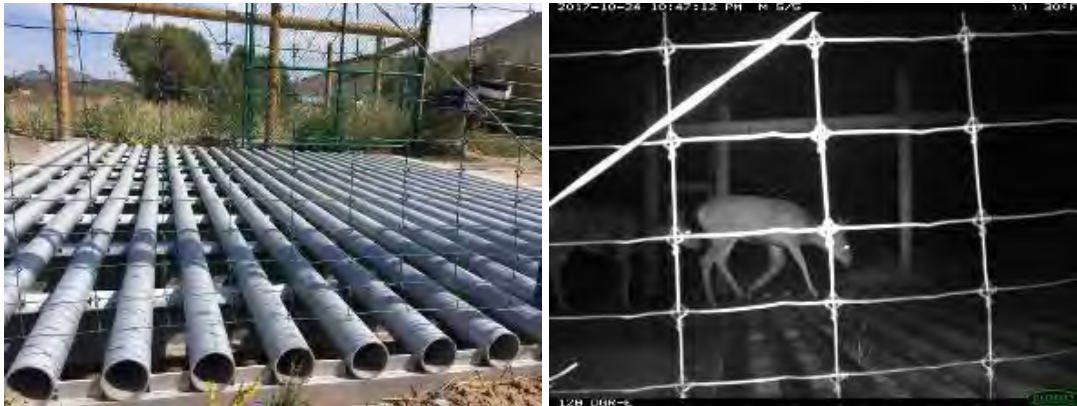
Figure D-45. Colorado SH 9 round bar double cattle guard (left) (photo credit: P. Cramer). How mule deer can use the support beams to breach the guard (right) (photo credit: CDOT, CPW, and ECO-Resolutions).
