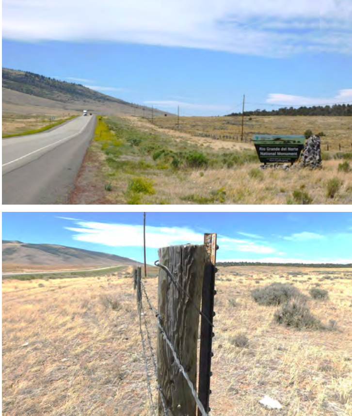
Figure 6-37. Rio Grande Del Norte National Monument and US 285 looking north (top) and Del Norte laydown fence in upright position (bottom) (photo credit: P. Cramer).
