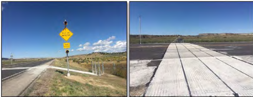
Figure D-58. Driver warning signs and electrified barrier at fence end on US 550, New Mexico (photo credit: AZGFD).
