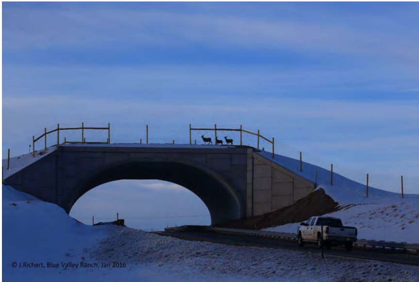
Figure 1-8. Mule deer moving over one of the SH 9 wildlife overpasses in Colorado (photo credit: Josh Richert, Blue Valley Ranch).
