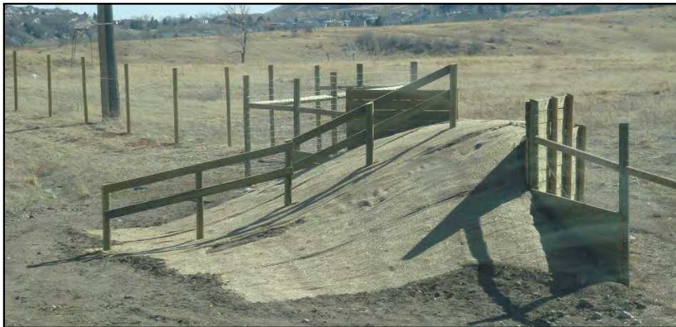
Figure 15. Escape Ramp Example
